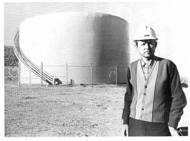
NEW AREA III water storage tank — 700,000 gallons — was completed recently. Earl Gruer (9742), Plant Engineering Department project engineer, reports that pumps and associated control equipment are being installed in the adjacent pump house and that the new water system should be in operation next week. The new tank, filled from a 10-inch line from Area I, serves primarily as a fire protection emergency system. It is positioned on a hill — elevation 5592 feet — on the south end of Area III.
